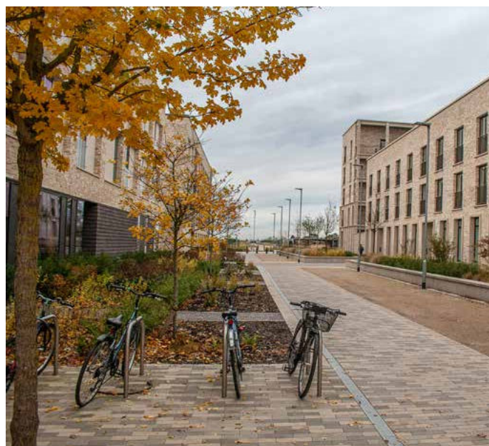
Top: Secure cycle parking integrated within a building (Chiswick Park, London)
